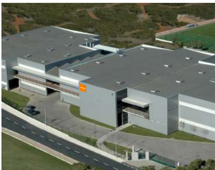
Wafer production and packaging buildings in Abóboda
